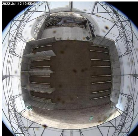
GRCF aerial snapshot of the tipping floor (top) and the bunker/aeration areas (bottom) before concrete was poured, showing the aeration piping embedded in the floor.
