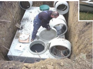
Replacing a septic tank and drain field
