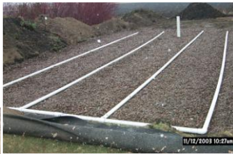
Replacing a septic tank and drain field
